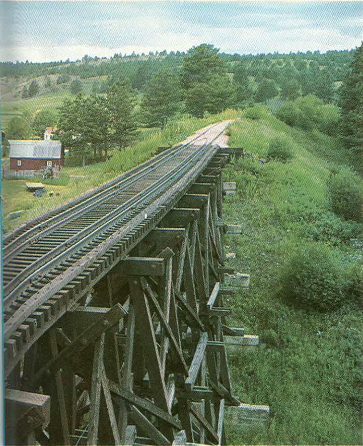
This abandoned stretch with its century-old trestles was laid in 1891 by the Chicago, Burlington & Quincy.
